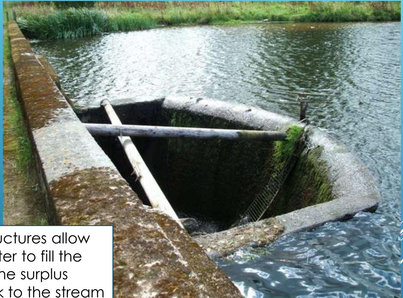
Overflow structures allow the fresh water to fill the ponds and the surplus to flow back to the stream
