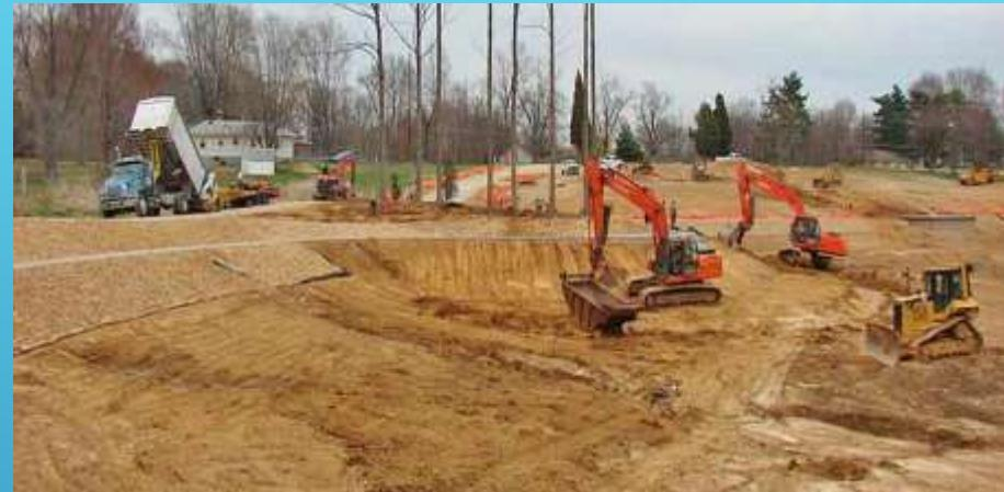
The ponds /lakes are constructed into the natural topography and are interconnected with naturalised streams and/or wetlands
