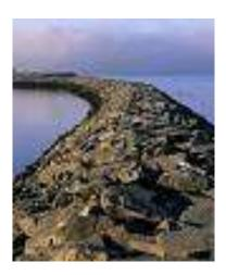
Rubble mound breakwaters use structural voids to dissipate the wave energy. Rock or concrete armour units on the outside of the structure absorb most of the energy, while gravels or sands prevent the wave energy's continuing through the breakwater core.
