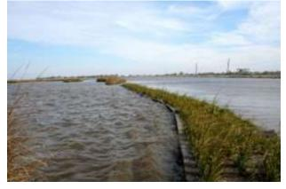
Synthetic rubberised bladders filled with sand are used in the Caribbean to provide safe swimming areas.
